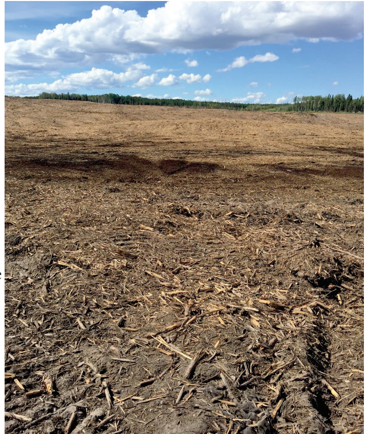
Completed fireguard with fuel (trees and bush) removed and/or mulched.
