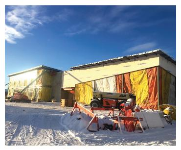
concrete floors decks, continuing with light gauge steel framing and roughing in for electrical, plumbing and HVAC.
